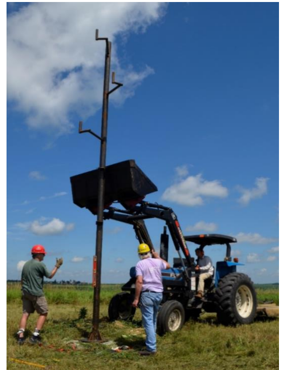
Erecting the Motus tower. Mark Martin
